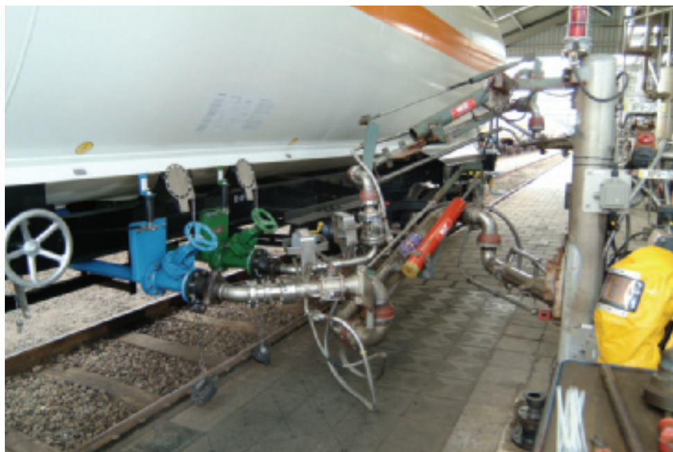
Figure 21 Typical lay-out of a loading/unloading arm with screw couplings
