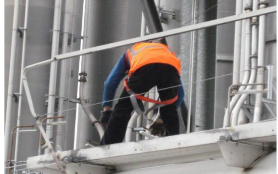
Harness not fitted correctly
