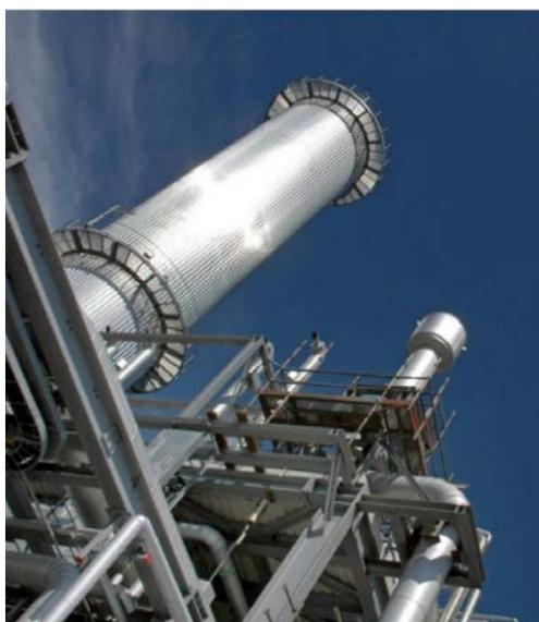
Chemical companies increasingly use combined heat and power (CHP) plants to generate both electricity and steam. Such cogeneration plants are an extremely effective means of supplying energy and, with an overall fuel efficiency of almost 90 percent, are the front-runners among energy conversion methods suitable for use on an industrial scale.
